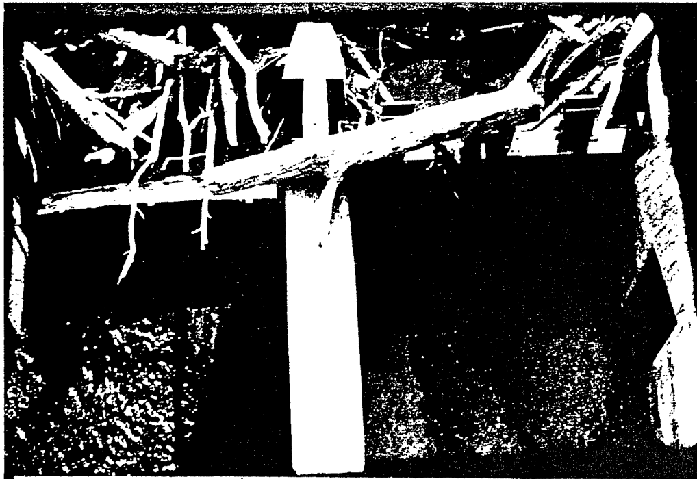
Picture 7 - Debris Buildup at Intake
