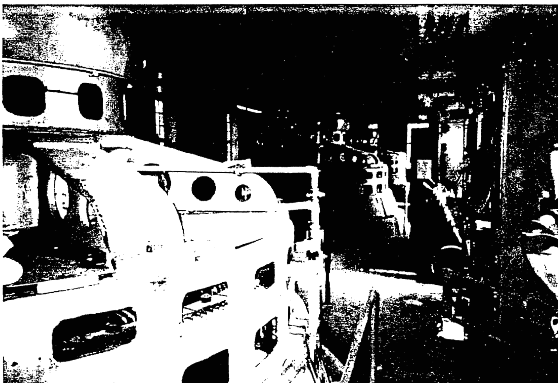
Picture #1 - View of Generators Looking from Unit 1
