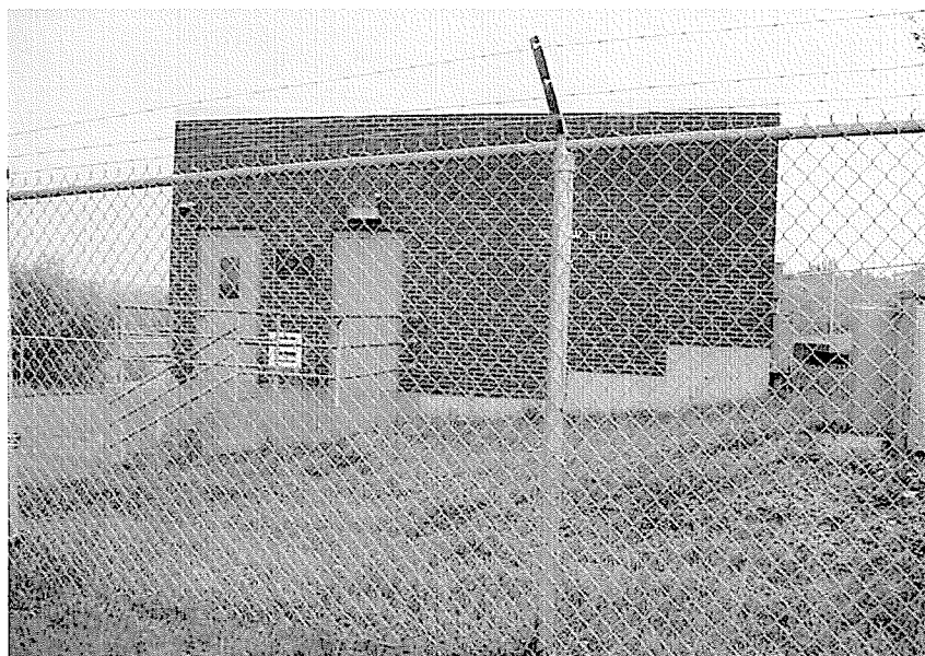
Ripple Creek Pump Station
