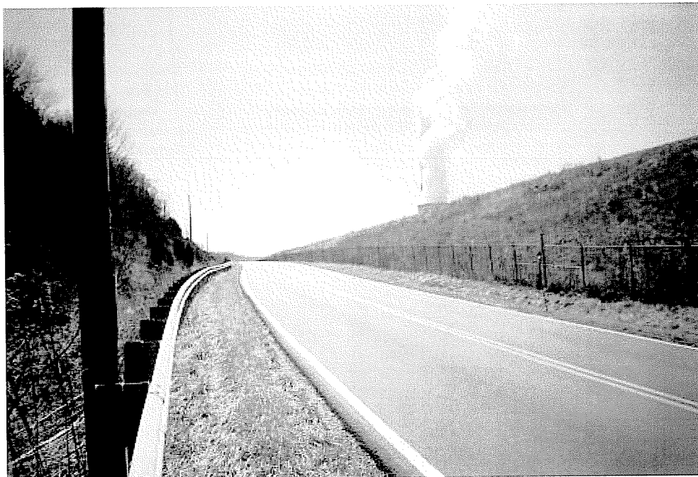
Figure B-4 View of Facility from P1
