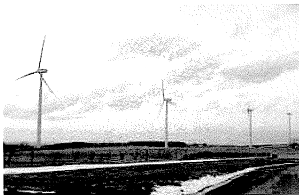
Figure 3-1. A 9 MW Wind Farm near Sommerset, Pennsylvania.
