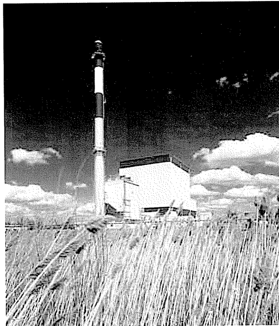
Figure 3-9. 35 MW Biomass Combustion Plant.
