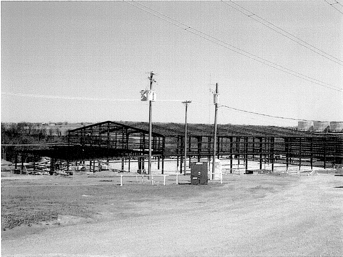
The above photo (dated 4/16/2007) shows construction of the new warehouse.
