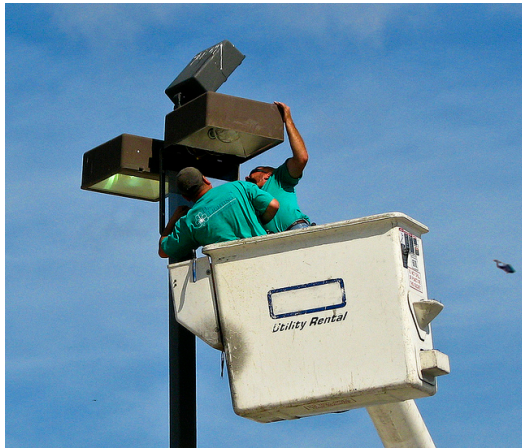
Figure 2-2. Replacement of lamps typically requires the use of a bucket truck, which can be costly
