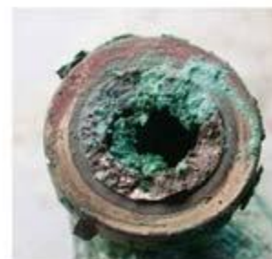
Corroded water pipe
