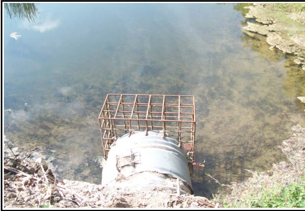
1) Inlet to the discharge pipe of the Hollybush Impoundment
