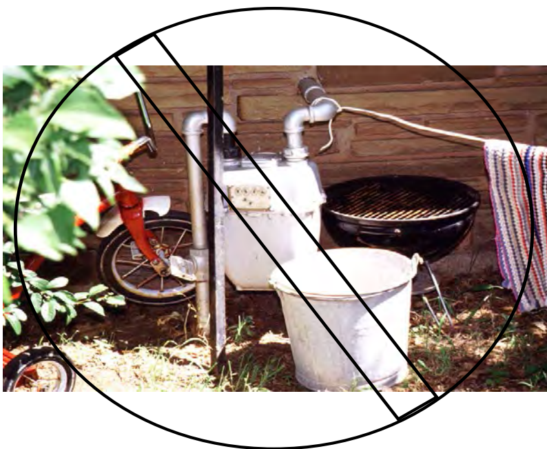
Figure III-15 Shorted Meter Set.
