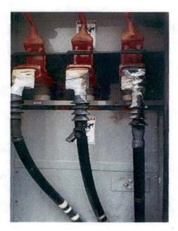
Photo 1. KU Substation initial cable fault on Cir. 45
