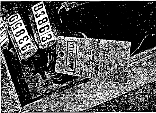
Pad Mount Transformer showing installed card and cable terminations
