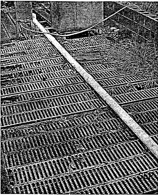
Preston Estates-Structural integrity of the grating needs to be checked
