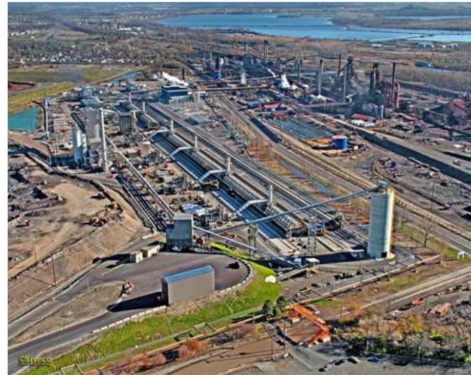
Heat recovery plant producing high quality steam and coke for neighboring steel mill
