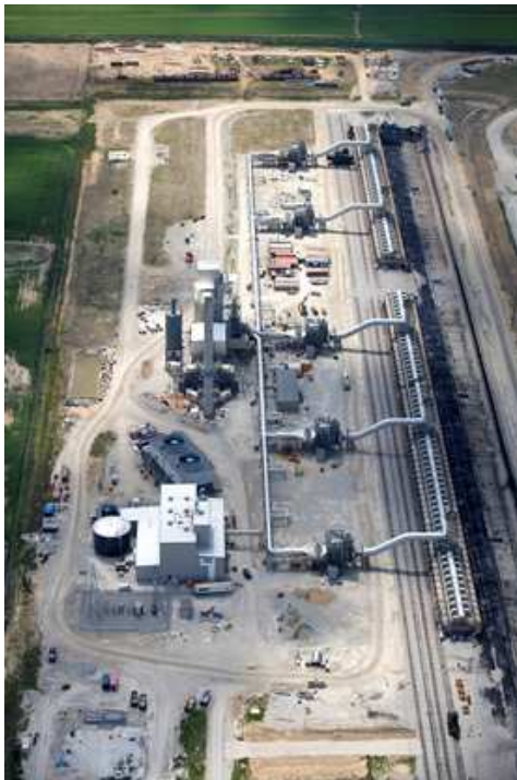
Expansion of existing plant with full heat recovery to power
