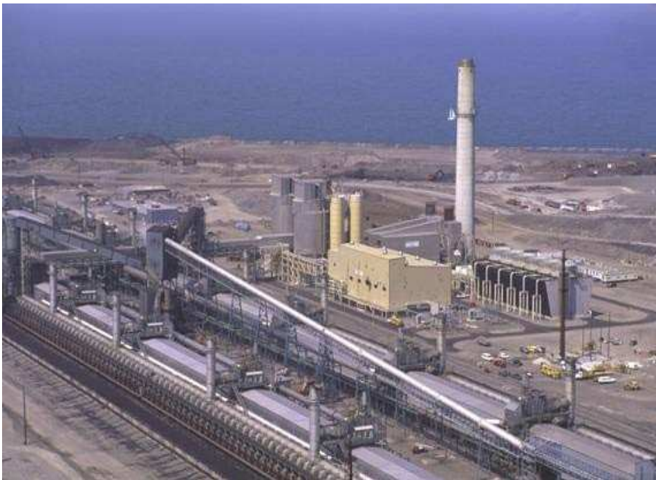
The first horizontal heat recovery coke plant in the US where waste heat generates steam to generate power, also includes flue gas desulfurization
