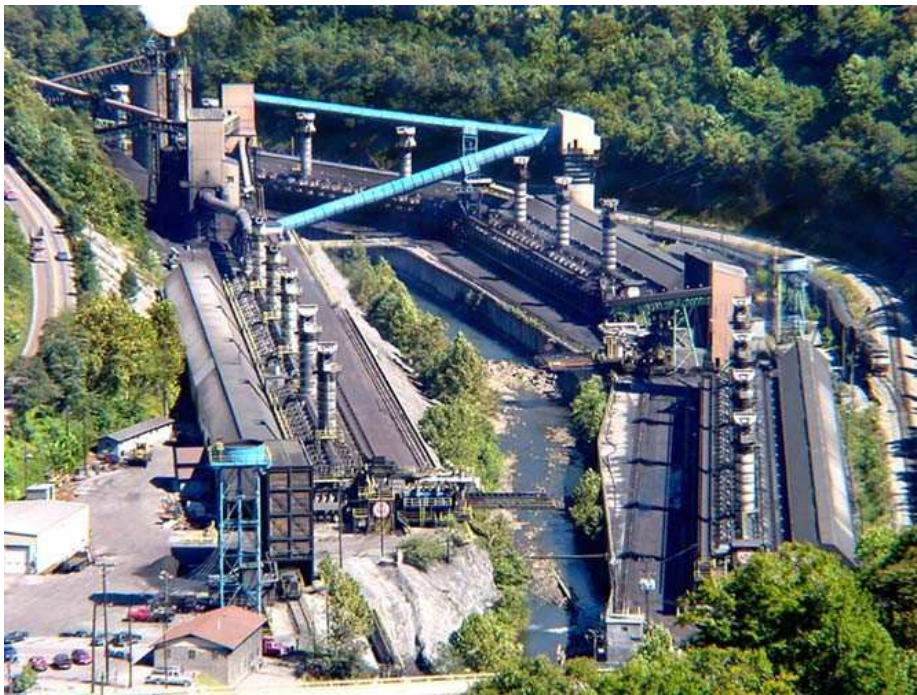
The first horizontal non-recovery coke plant in North America, a portion of the flue gas is used to dry coal
