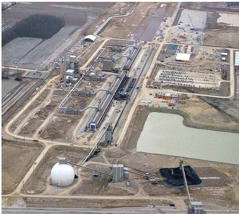
The first of the current generation heat recovery coke plants supplying plant steam to a nearby chemical plant
