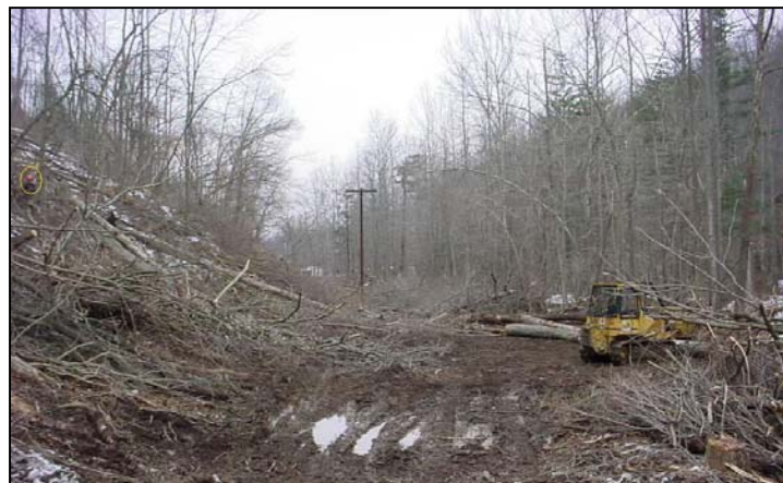
PHOTO 14: Lewis County, KY ~ Bulldozer Clearing R/W
