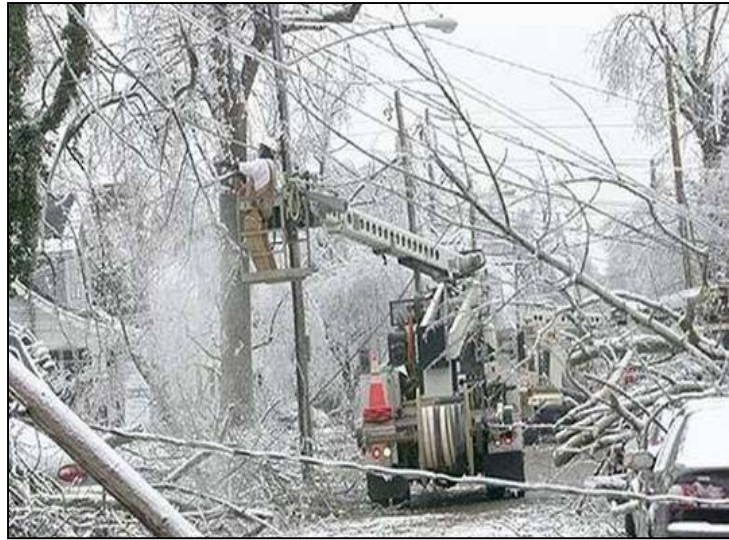
PHOTO 9: Alltel Repair Crew ~ Lexington, KY
