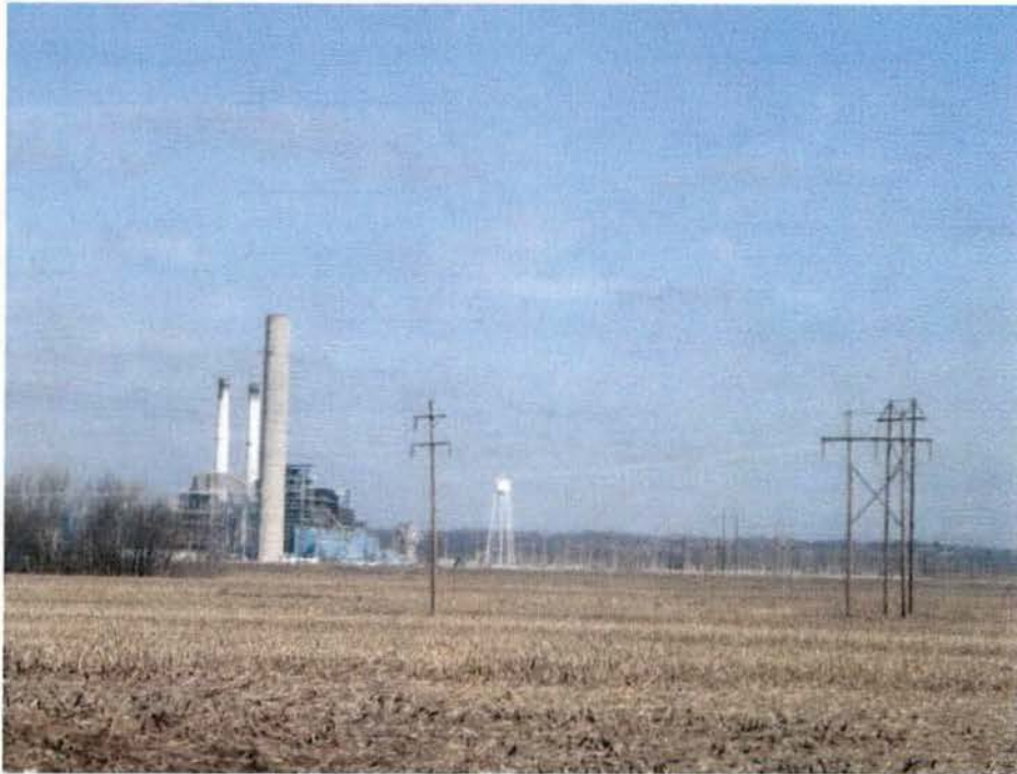
PHOTO: Existing Transmission Line in Hancock County
