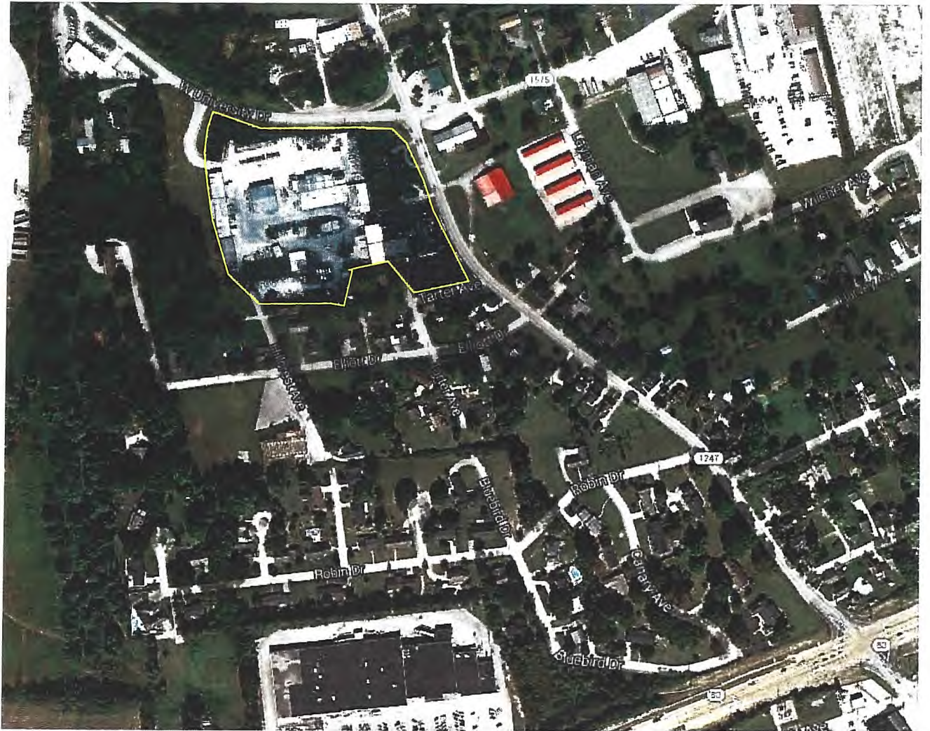
South Kentucky RECC (Pulaski Co.) Existing Headquarters
