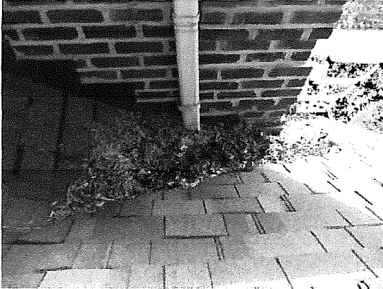
please monitor the valleys for debris accumulation
