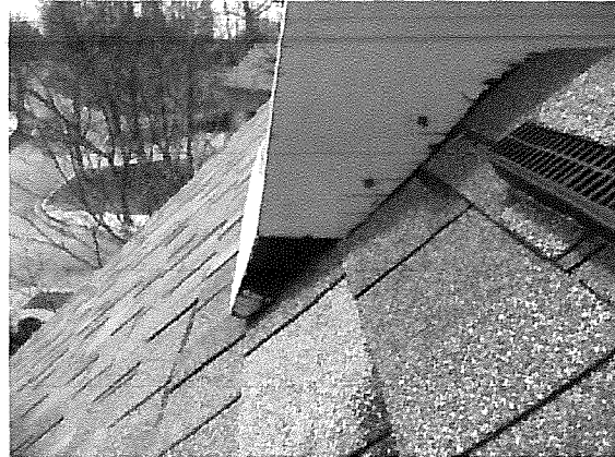
opening at the back side of the cupola should be sealed to help prevent pest entry
