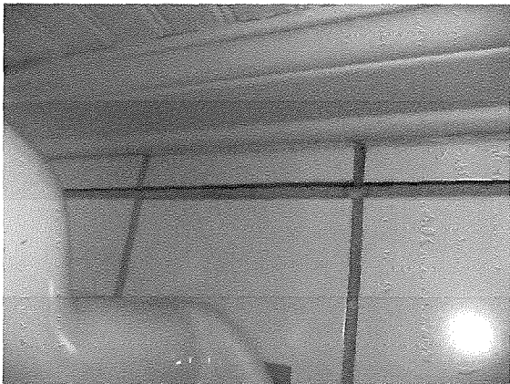
second level jack-n-jill bathroom tile behind the commode
