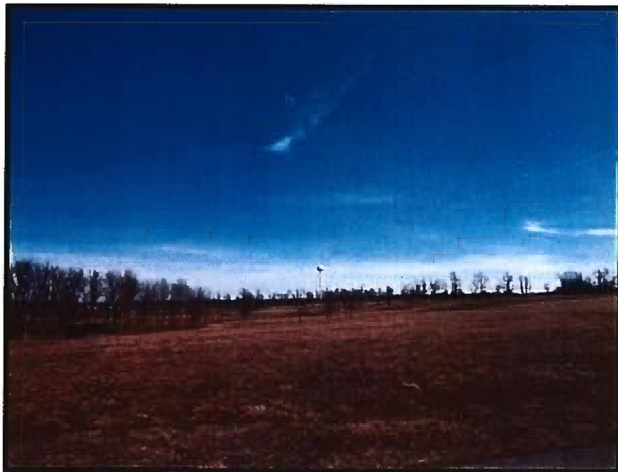
View of 50KG Tank From Eagle Drive
