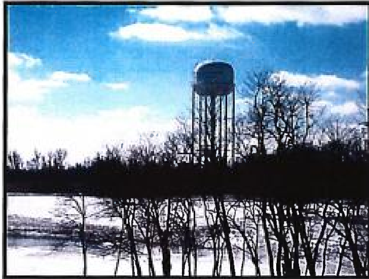
View of 500KG tank Behind 302 Eagle Drive
