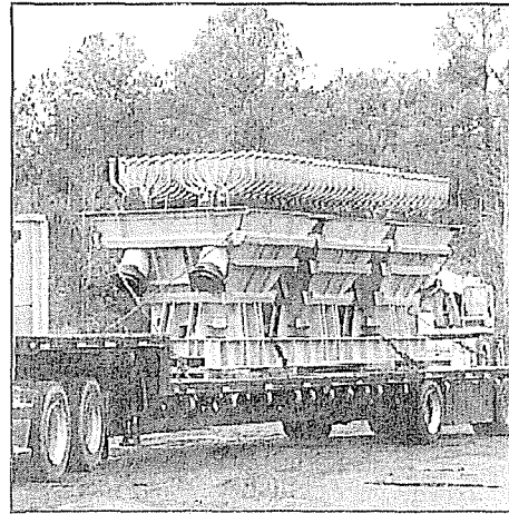
Bed hopper modules reduce erection time
