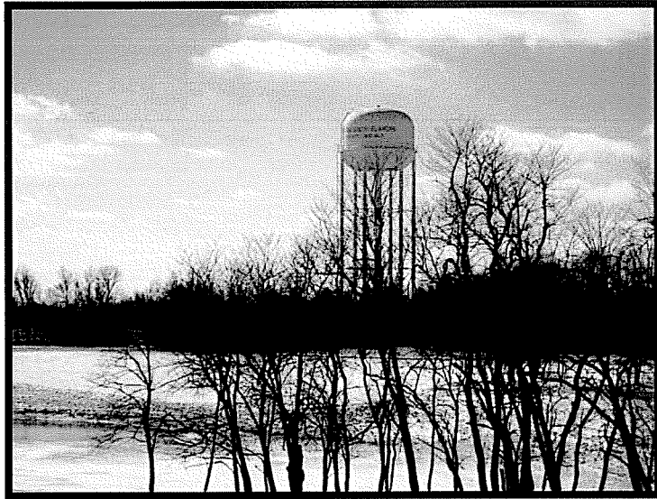
View of 500KG tank Behind 302 Eagle Drive
