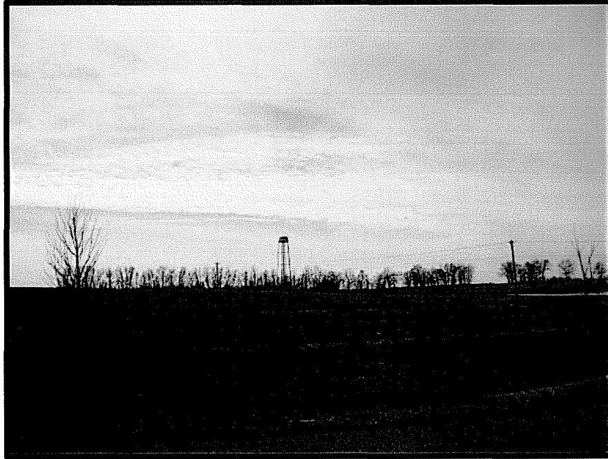
View of Existing 50KG Tank @ Entrance to Forest Hills
